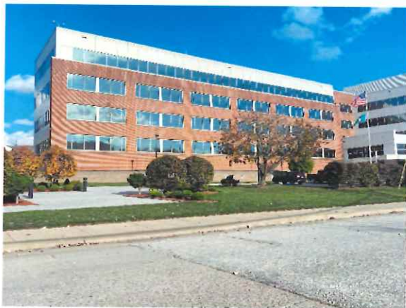
Figure 48: Fiscal Services Building
