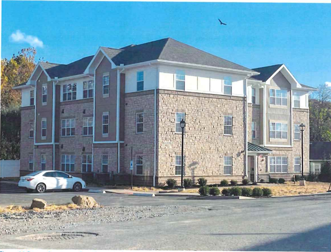
Figure 44: Rowan Apartment Complex on Buckeye Street
