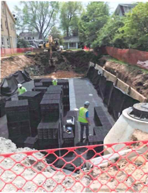
Figure 39: 20 th Street Stormwater Retention Project
